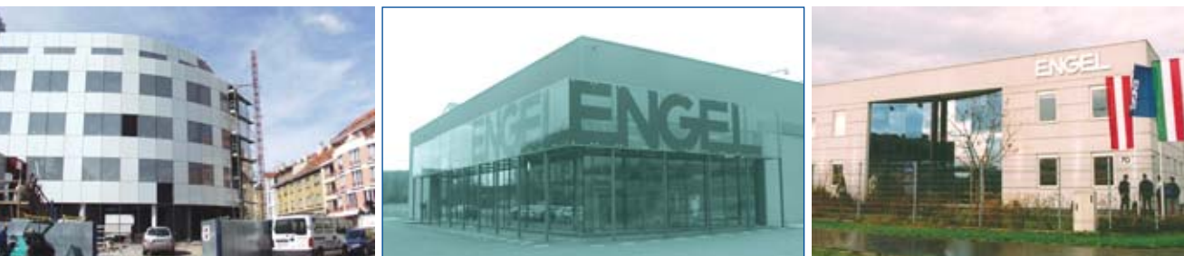
Left: Engel Czech Republic will move into its new building in Prague at the end of 2005. Centre: The planned building of Engel Poland in Warsaw will be completed by the end of 2006. Right: Engel Hungary has been in its new building in Budapest since November 2002.
